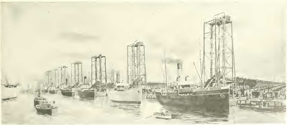
Hydraulic Coal Hoists at the King's Dock Immingham.
